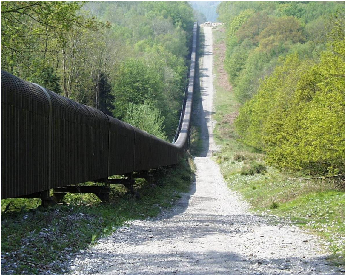
Fig 5. The Brightling Mine to Robertsbridge overland curved conveyor installed in 1986.
