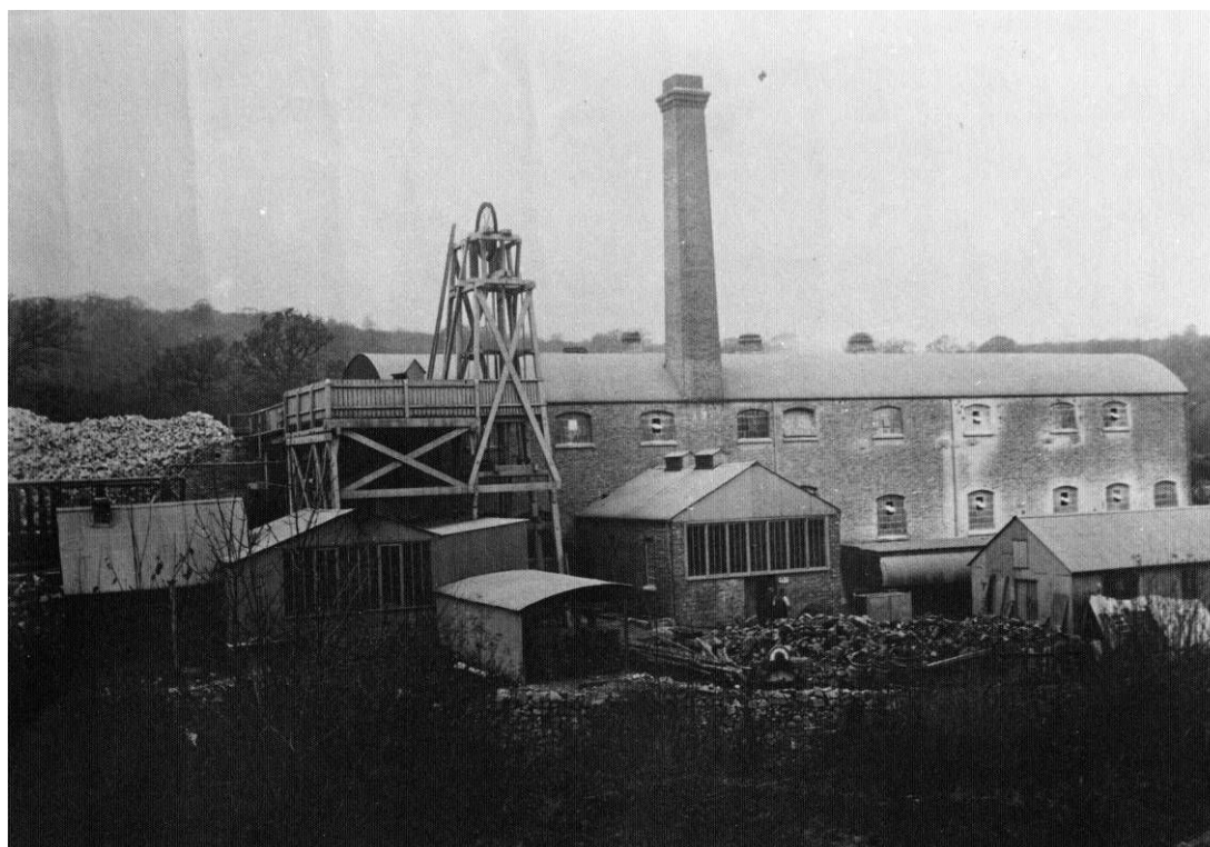
Fig 2. Mountfield Mine and plaster works in the late 19 th century. The Woodland Shaft some 45m deep was used to raise gypsum to the surface.
